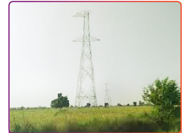
765kV Ghatampur TPS-Agra SC line
