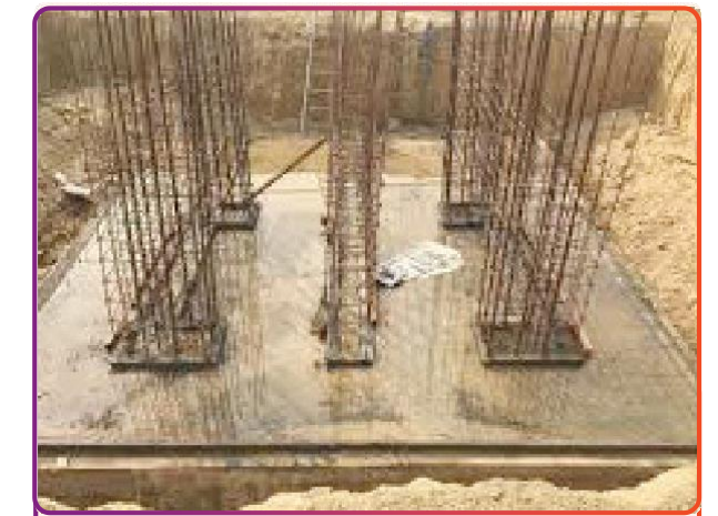
160 MVA ICT-2 foundation work at Badaun Sub-station (Obra line)
