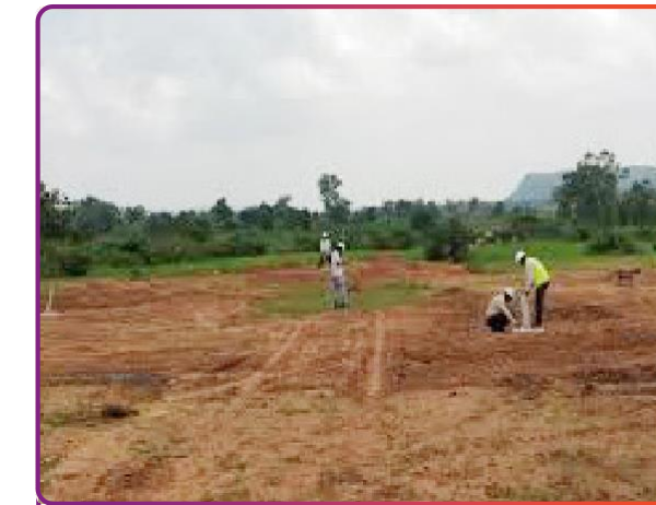
Completion of tower foundation work at North Karanpura-Chandwa (NKTL)
