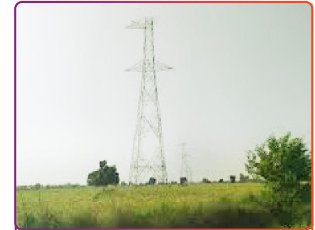
765kV Ghatampur TPS-Agra SC line
