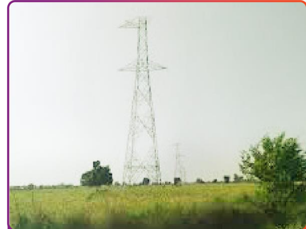
765kV Ghatampur TPS-Agra SC line
