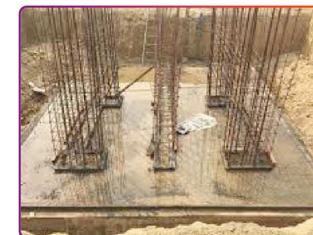
160 MVA ICT-2 foundation work at Badaun Sub-station (Obra line)
