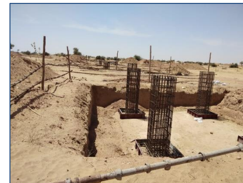
400 kV pooling station work at Fatehgarh 2 (FBTL Line)
