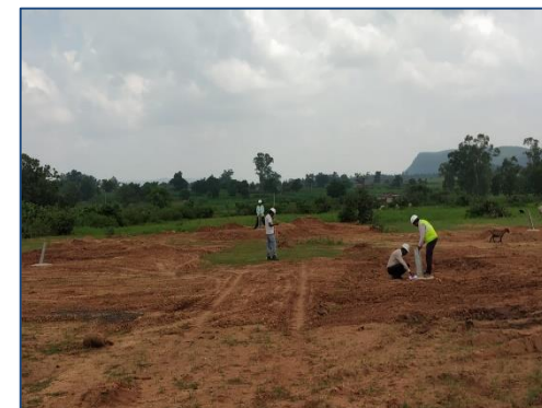
Completion of tower foundation work at North Karanpura-Chandwa (NKTL)
