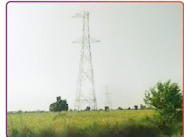
765kV Ghatampur TPS-Agra SC line
