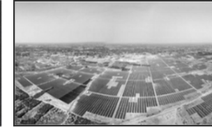
648 MW Ultra Mega Solar Power Plant
