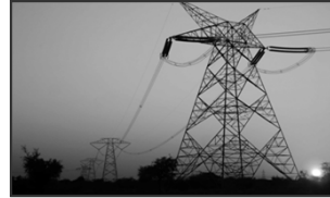
Longest Private HVDC Line in Asia
