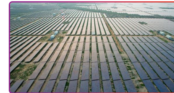
648 MW Ultra Mega Solar Power Plant (at Kamuthi, Tamil Nadu)
