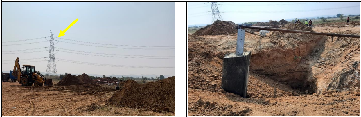
Photo 7. Ongoing Tower Foundation Work (Existing PowerGrid Transmission Line )
