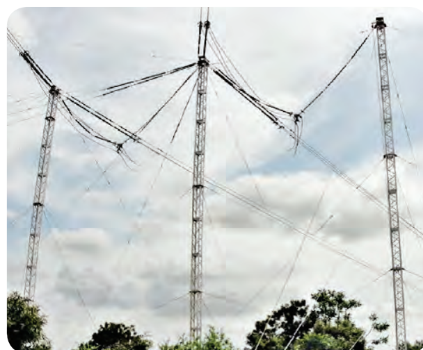
> HVDC line erected on the ERS
