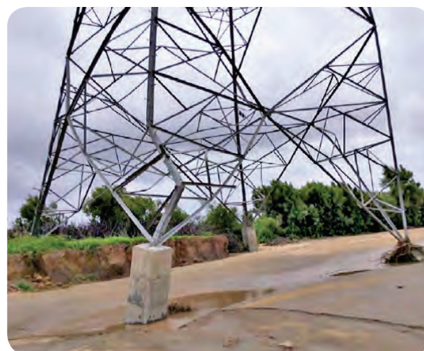
> Damaged foundation of the tower
