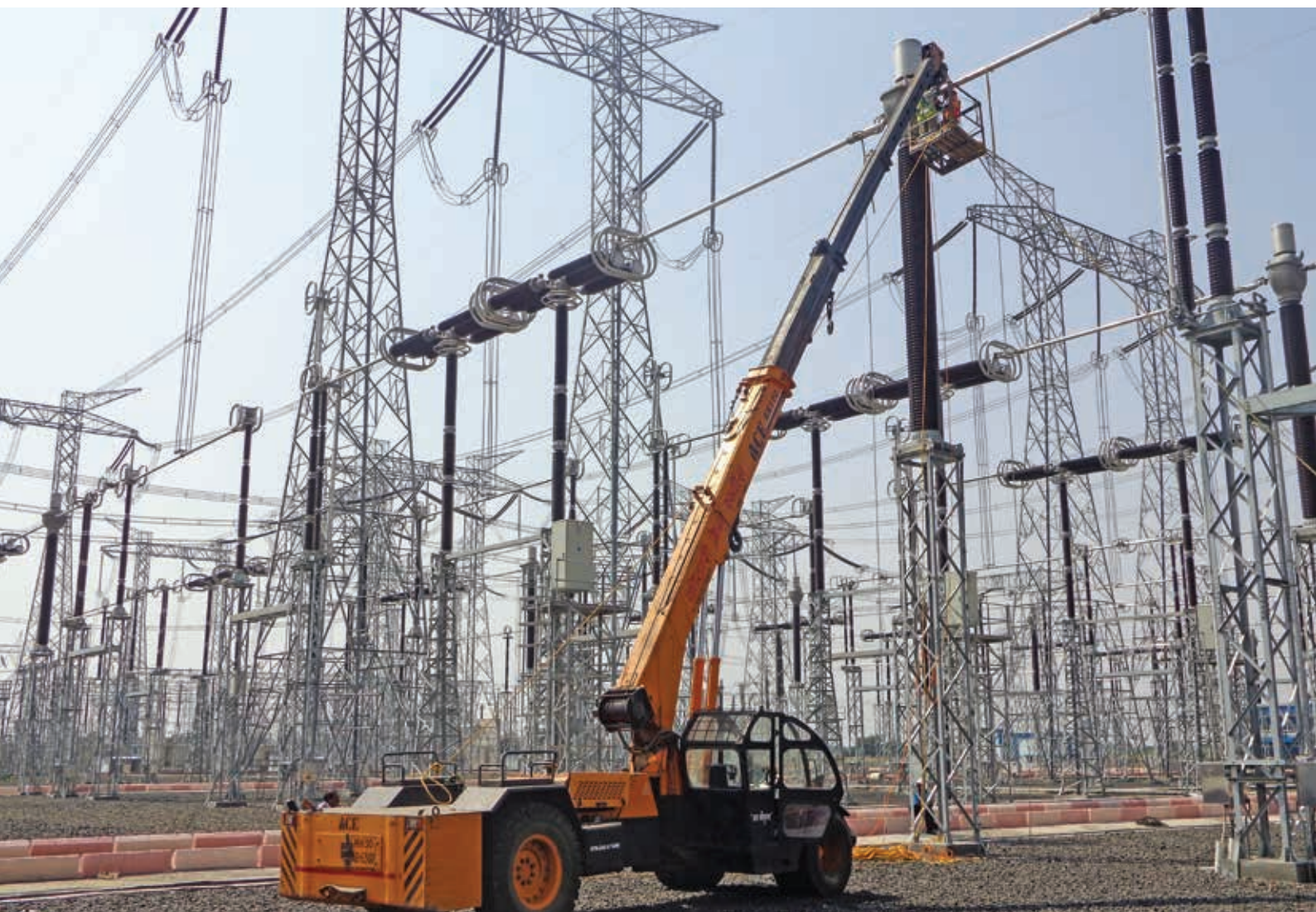
Current Transformer (CT) maintenance work in progress at 765 kV Koradi substation.
