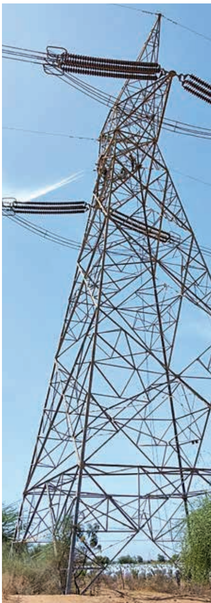
Performing Hot Line Washing of Insulators
