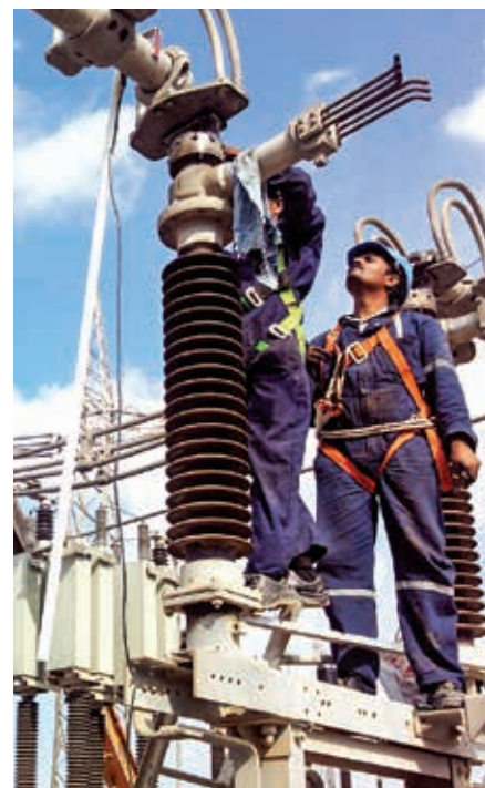
Isolator maintenance work in progress at ± 500 kV HVDC Mundra substation
