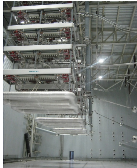
Fig. HVDC Valve Hall
