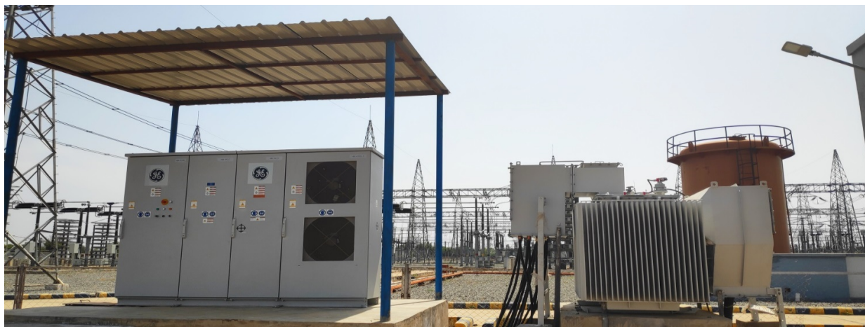
APFC Panel and Transformer
